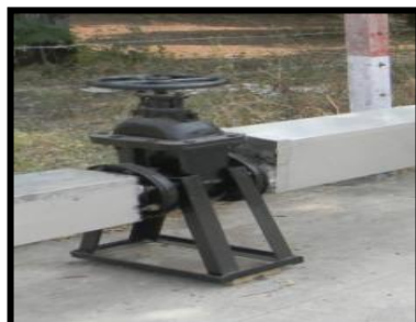
Plate 3: Wheel valve (6"Ø)
