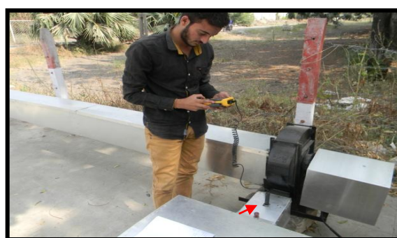
Port 3 between blower unit and heating box
