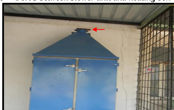
Port 5 at the top of drying chamber (exhaust end)
